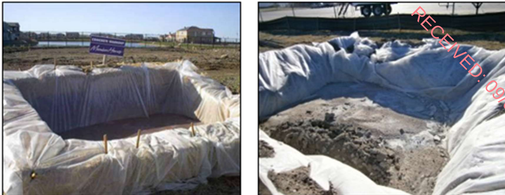
Plate 3-1 Typical concrete wash out areas
